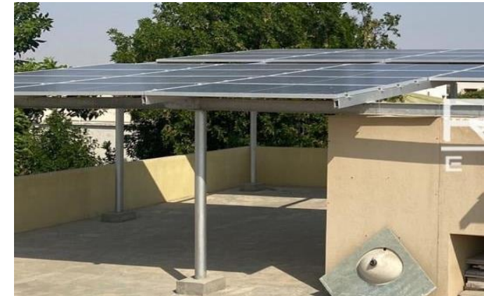
Hot Dip Galvanized Elevated Structure
