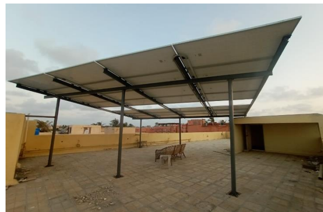
H-I Beam Elevated Structure
